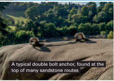
Always use non-stretch rope or slings to extend your anchor over the crag edge and avoid moving rope contacting the rock
